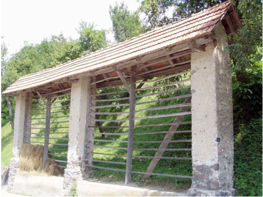
Figure 3. Enojni stegnjeni kozolec z zidanimi stebri. Cerčno, Slovenia. Photograph by Author.
